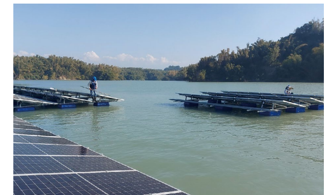
Modules are being moved to their positions
